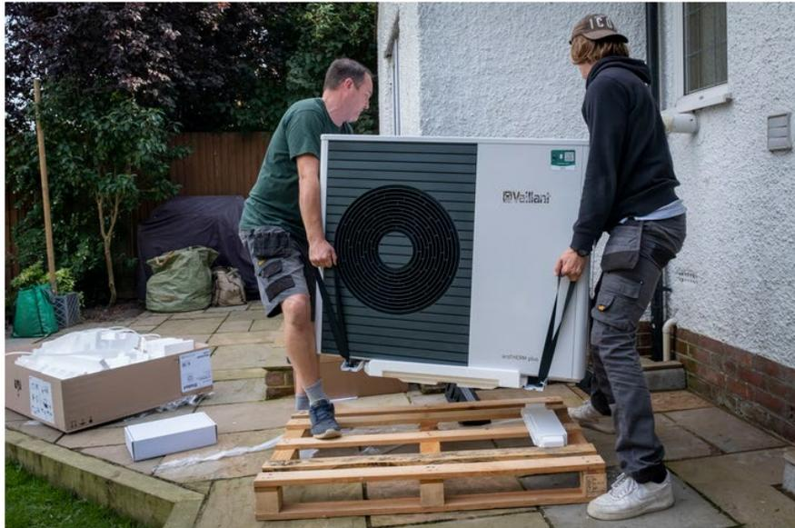
This Machine Fights Fascism (an air source heat pump being installed last September in a house built in the 1930s in Folkestone, UK).
