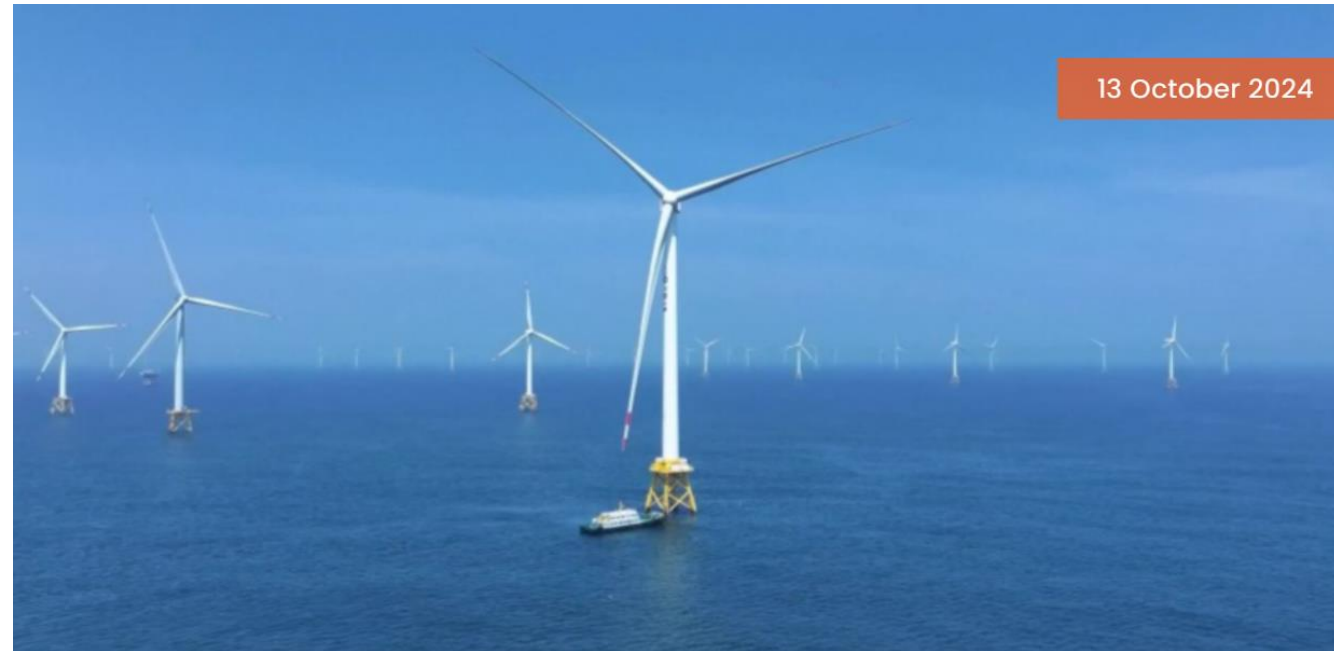
26-MW Turbine offshore, 310 diameter !
